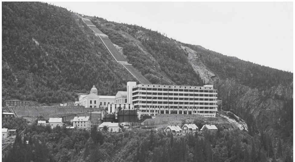
The Vemork power station at the Rjukan Falls was the world's largest hydroelectrical power plant when it opened in 1911. Photo: Anders Beer Wilse / Norsk folkemuseum
